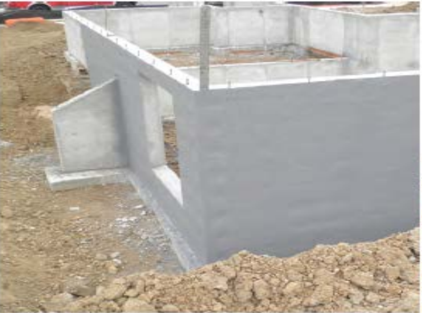
Footing–basement wall
